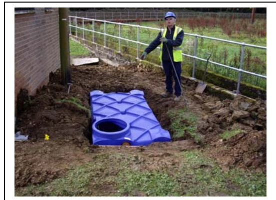
Simple rectangular hole Minimum excavation - approx 3m 3
