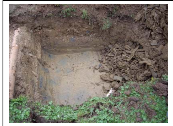
Simple rectangular hole Minimum excavation - approx 3m 3
