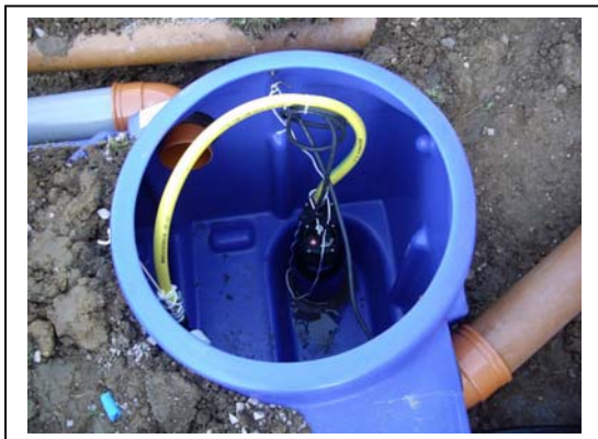
Pump (self priming) fitted with water connection Inflow/overflow and service ducts connected
