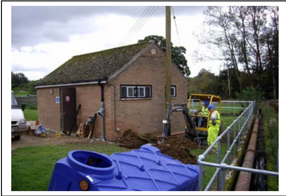
Downpipe filters fitted Flat Tank Excavation - approx. 1 m deep
