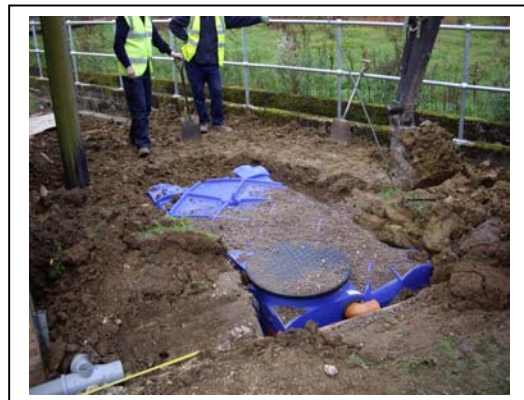
Backfill material surrounding tank completes installation
